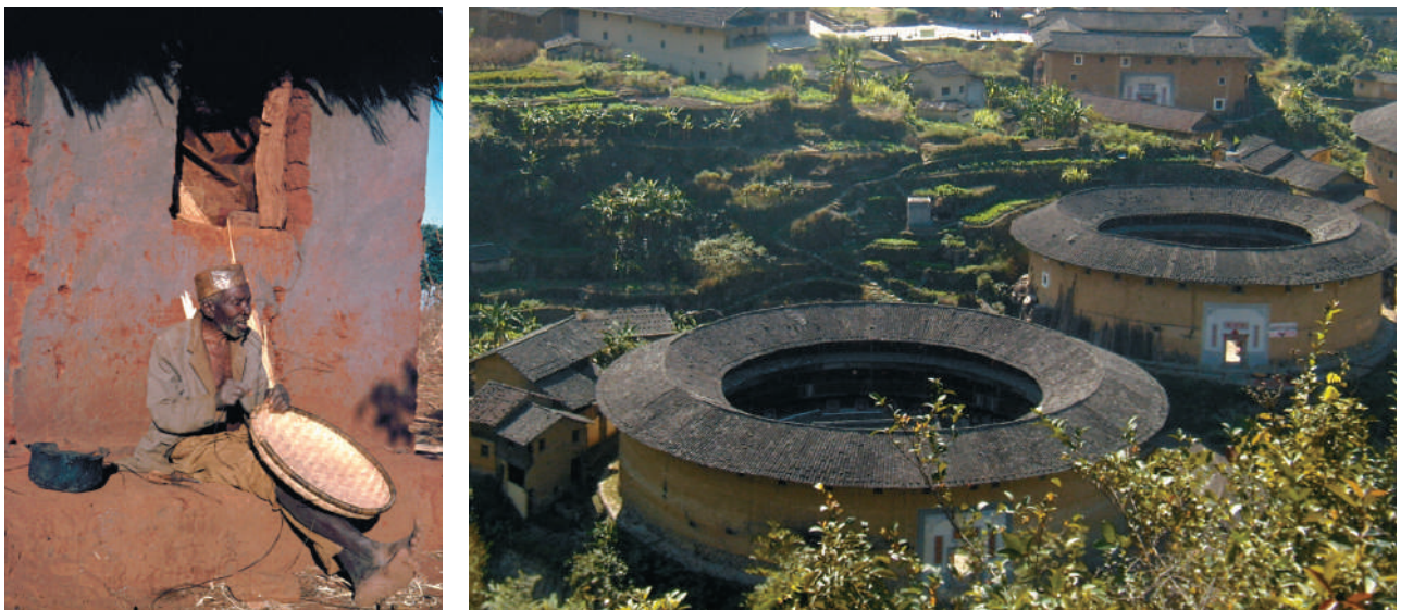
Figure 1.10 Soil is among the oldest and most common of building materials, with half the world's people living in homes made of soil. (left) An elderly African villager weaves a basket outside his house made from red and black clay soil reinforced with small tree branches (a technique termed wattle and daub). (right) Several round Tulou apartment buildings housing up to 80 families each in Fu-Jian, China. These buildings have 2-m-thick walls made thousands of years ago from compacted yellowish soil mixed with bamboo and stones. These massive "rammed earth" walls make the buildings warm in winter but cool in summer (see Chapter 7) and resistant to damage from earthquakes. (Left photo courtesy of Ray R. Weil; right photo courtesy of Lu Zhang, Zhejiang, China)
